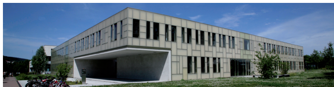
Façade with LAMILUX Façade Panel sheets
